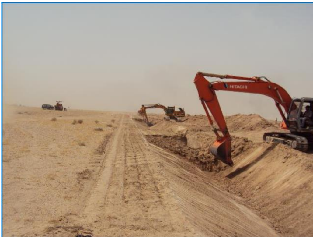
Ditch and Berm construction at Rumilla oil field
